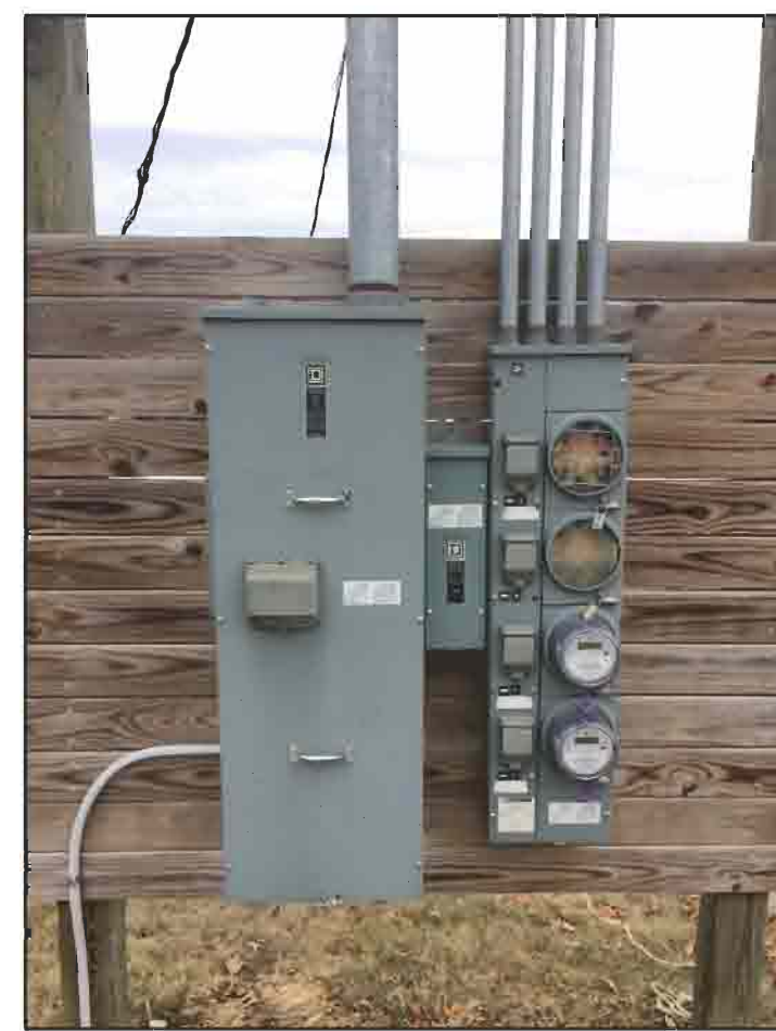
EXISTING (4) METER PAK - OVERHEAD SERVICES SCALE: NTS
