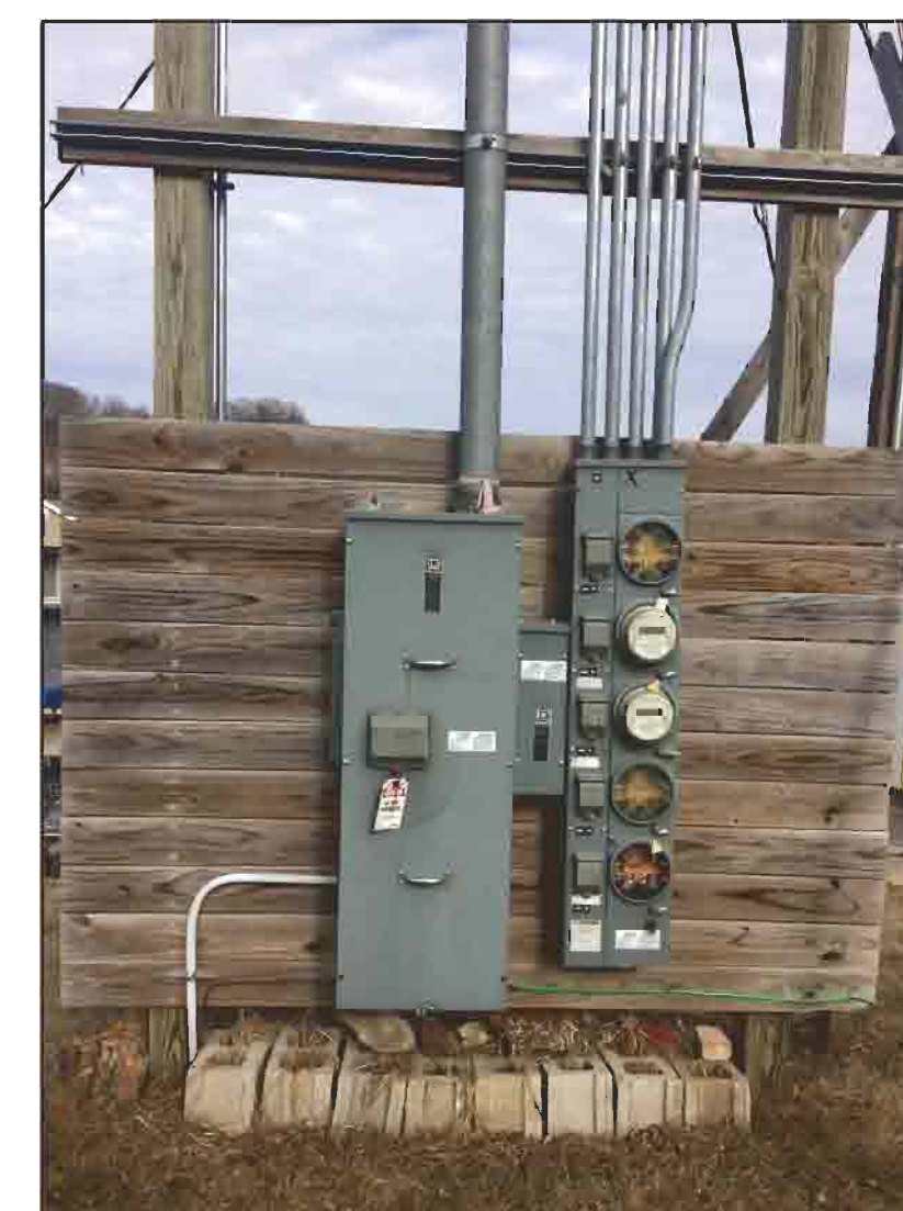
EXISTING (5) METER PAK - OVERHEAD SERVICES SCALE: NTS
