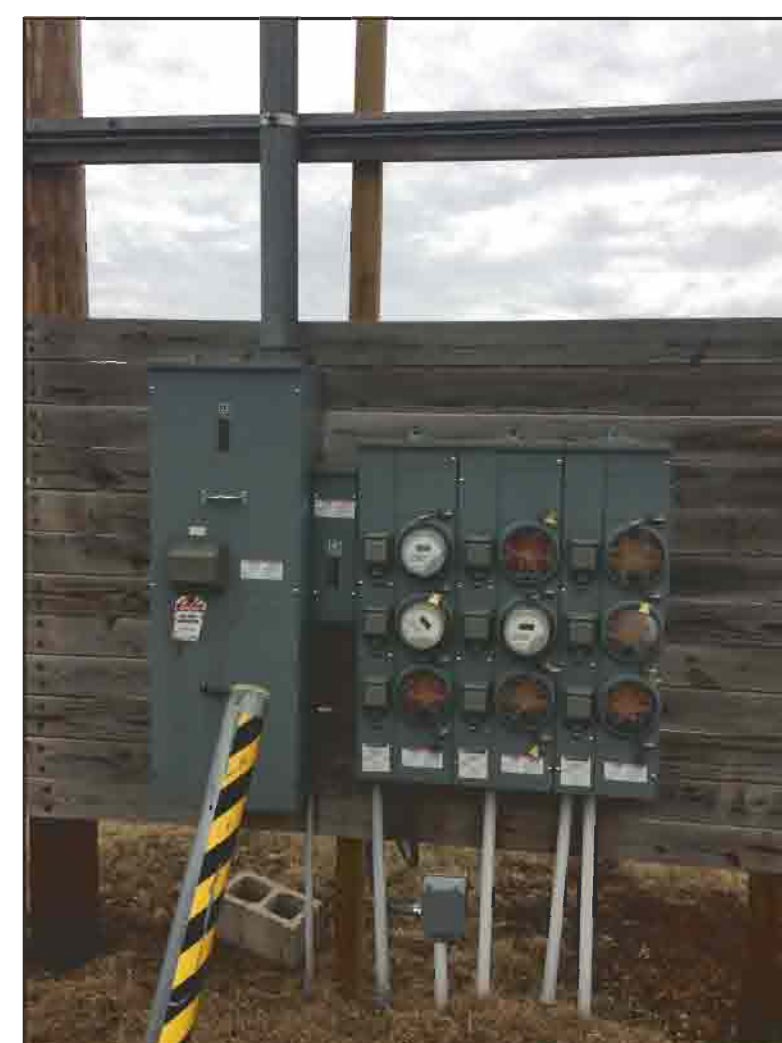
EXISTING (9) METER PAK - UNDERGROUND SERVICES SCALE: NTS
