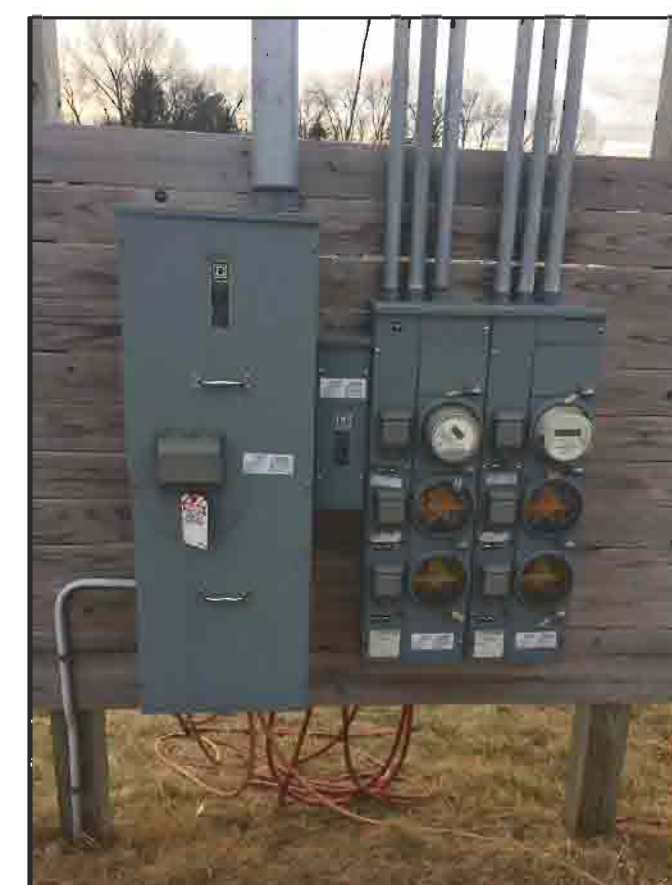
EXISTING (6) METER PAK - OVERHEAD SERVICES SCALE: NTS
